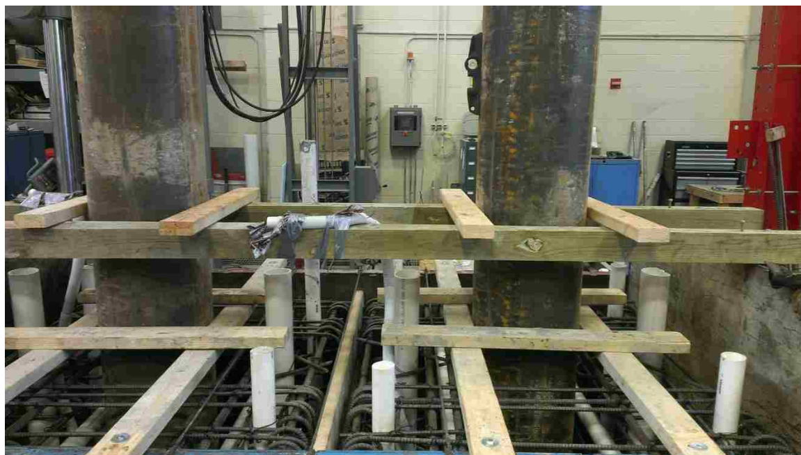
Figure B.6. Fixing the steel tube before pouring the footing
