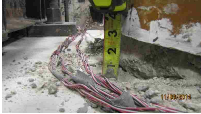
Fig. 9. Joint opening of the F4-24-E324 column at lateral drift of 14.1%
