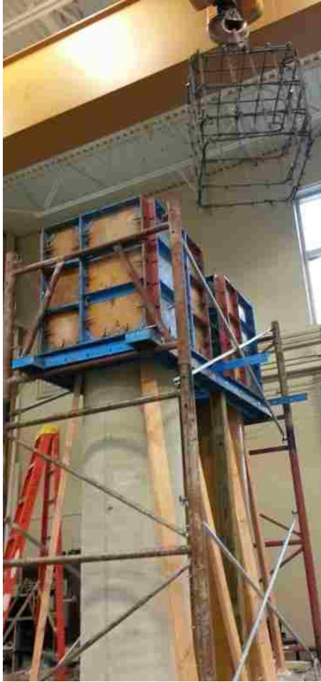
Install reinforcement cage
