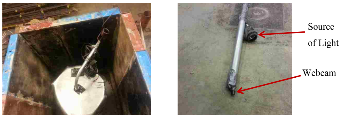
Figure B.16. Install webcams inside the steel tubes
