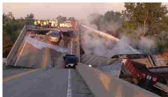
Figure 2.8. Trains accident-overpass outside of Scott City, Missouri, 2013 (McGrath 2013)
